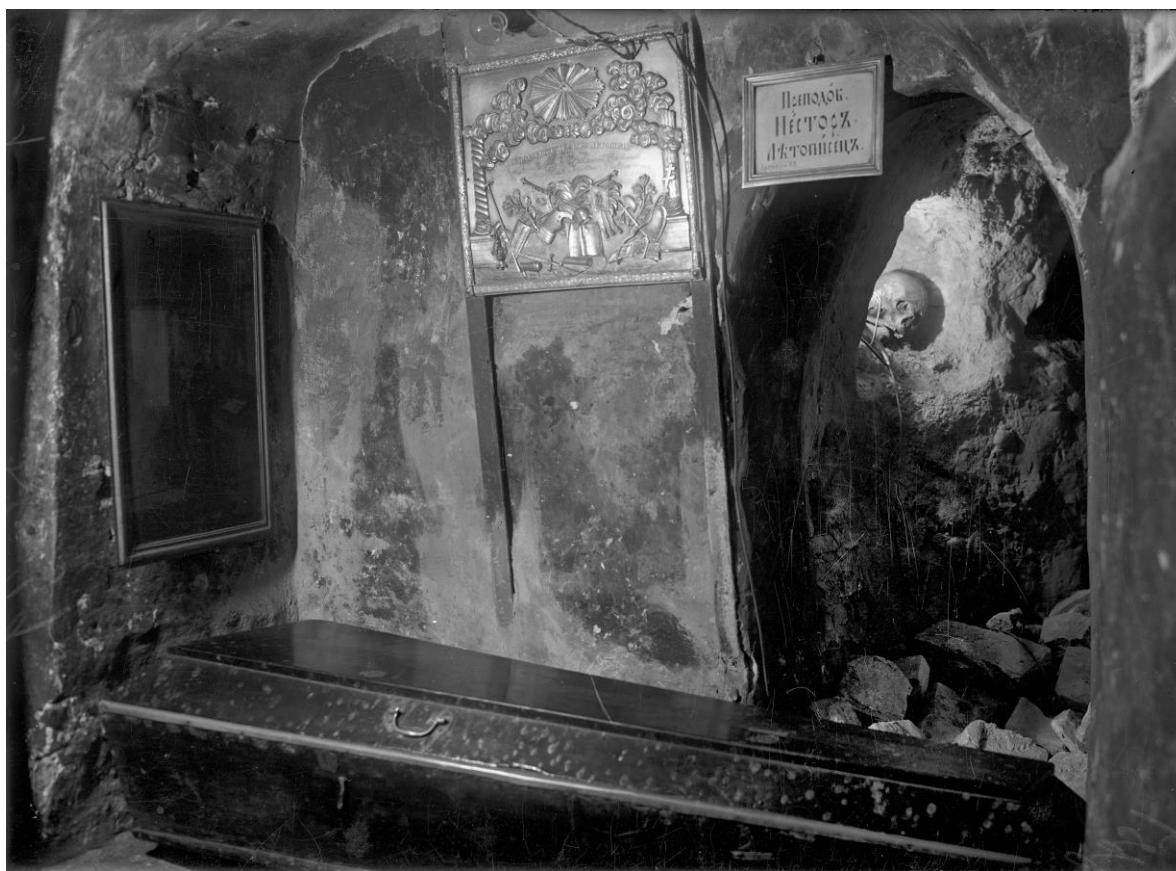
Fig. 6 The dismantling of the wall – the revealed walled cave passage – near the shrine (coffin) with the relics of holy righteous Nestor the Chronicler. 1934? (KPL-N-1371)
